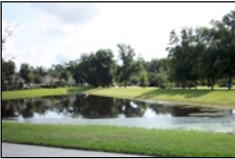
An example of the type of retention area now required for subdivisions to prevent run-off (Source:USF)
